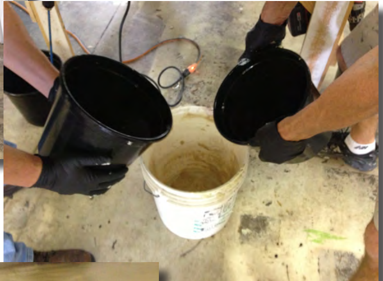
Right: Equal parts of the two part mixture are combined and mixed.
